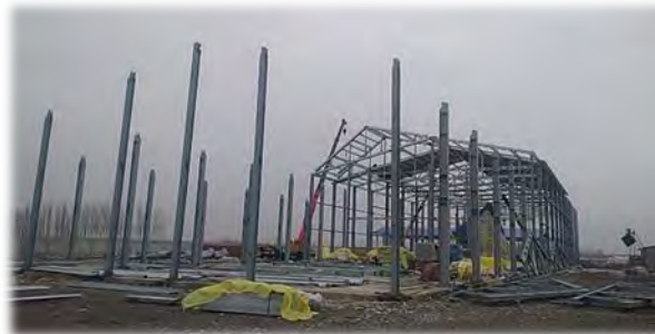
A large industrial building under construction, showing the steel framework and roof structure. The building has a high, vaulted roof and is surrounded by construction equipment and materials.
